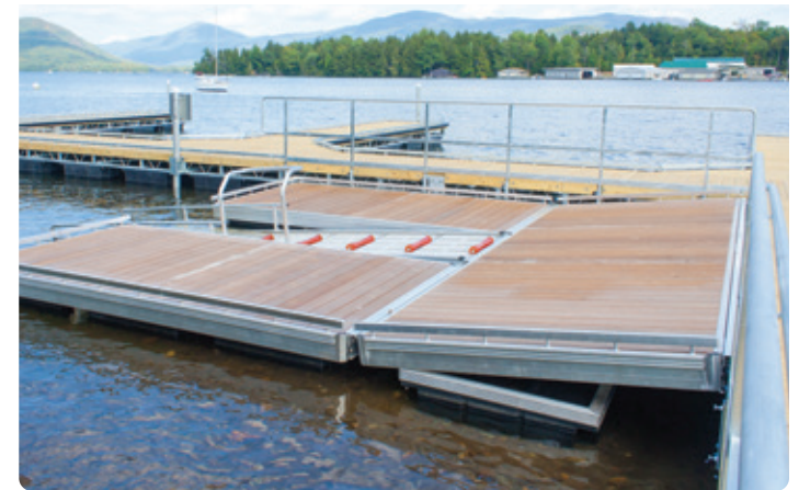
Hinge & connection at top of ramp to our galvanized steel truss floating dock.
