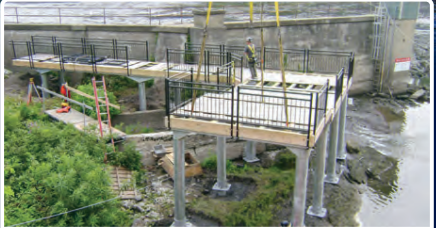
Installation of an industrial access platform at a hydro-power plant on the Mohawk River (Note: water level was lowered to facilitate installation).
