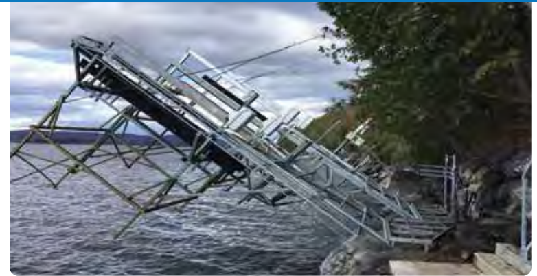
Above: Our Ultimate Lift customized to attach to the shore with galvanized lift arms allowing it to be raised for winter storage.
