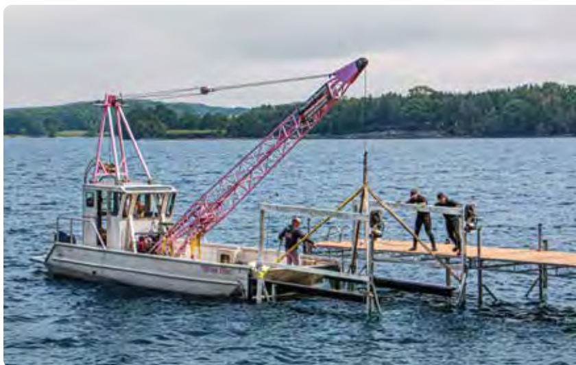
Above Left: 6000 lb. capacity Ultimate Lift being installed with our workboat "Miss Doc" and service crew.
