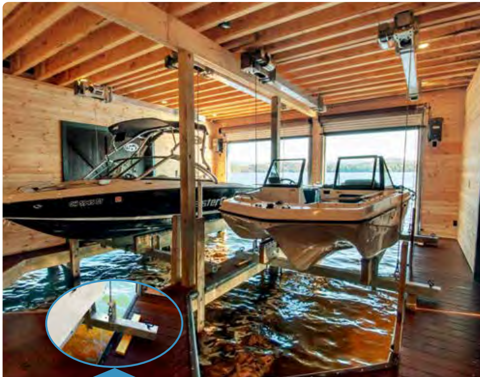
Bunk-style cradle system with pull-out tubes in place for winter storage.
