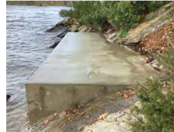
Top: L-shaped articulating dock with a concrete pad as a shore anchor.
