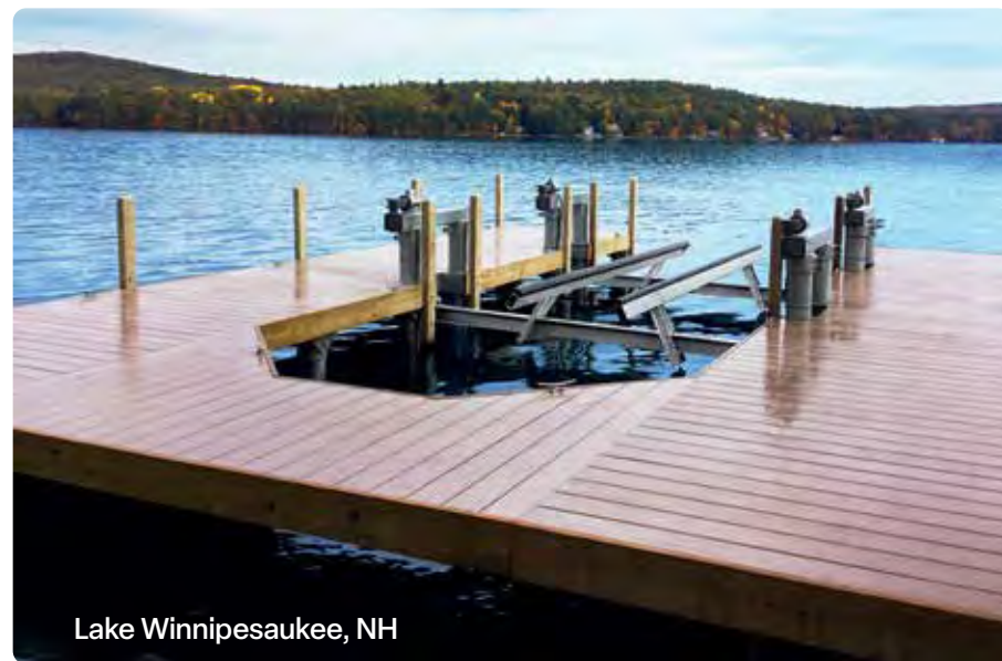
Custom 12,000 lb. hot dipped galvanized steel boat lift incorporated into the pile dock framework in order to maximize the slip width for the customers boat.
