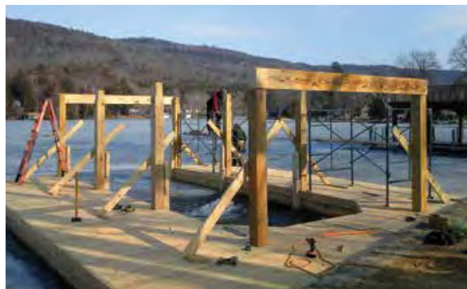
Cribs completed and boathouse structure in progress.
