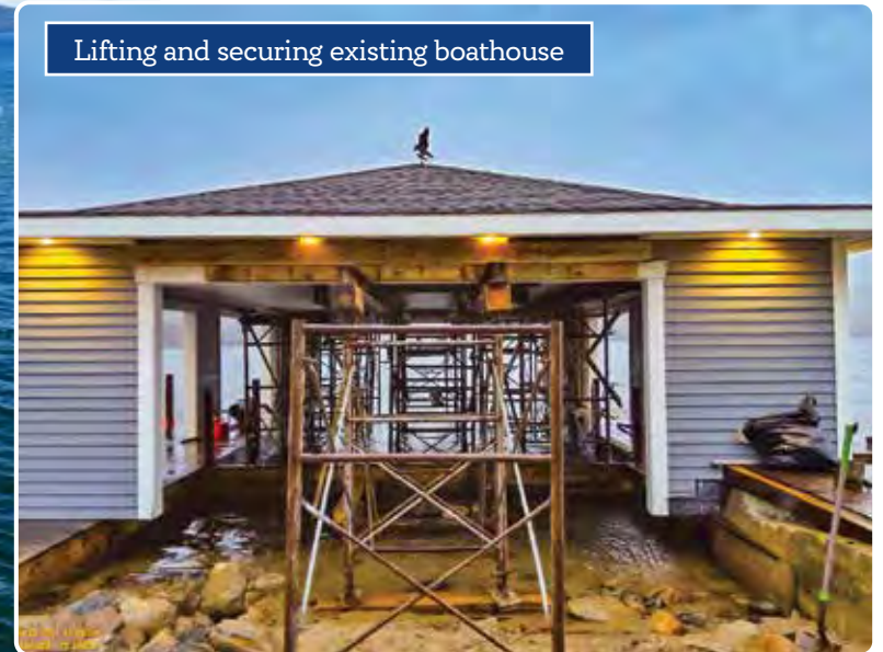
Above: New boathouse foundation complete. Above Right: Lifting and securing the existing boathouse to install new pile dock.
