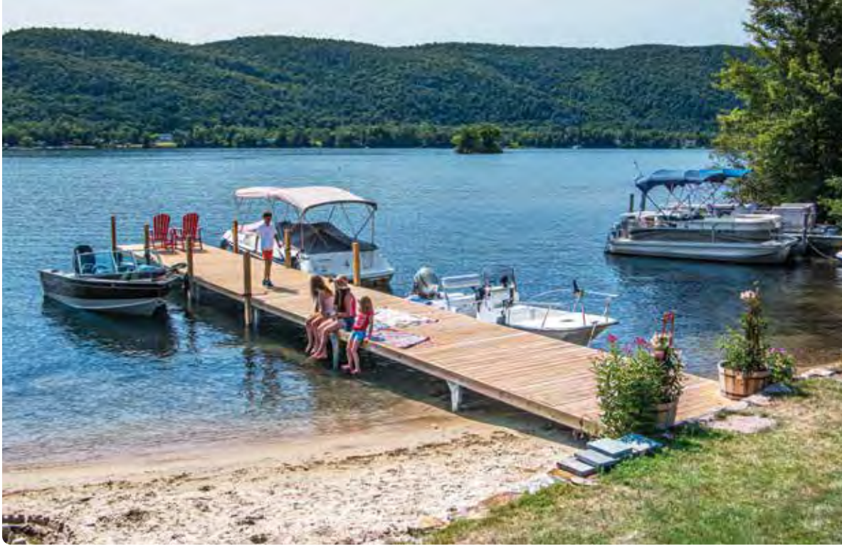
Above: Pile dock with rub strakes and piles cut below the decking.
