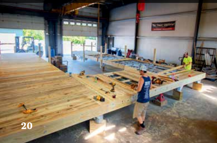
Final decking being applied in our workshop.
