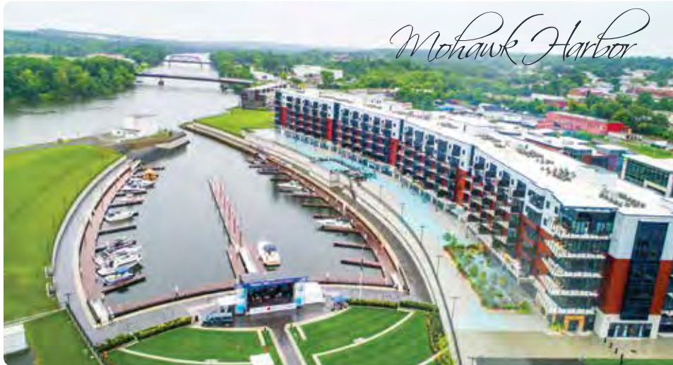
Commercial Marina Floating Dock System Mohawk Harbor, Schenectady, NY
