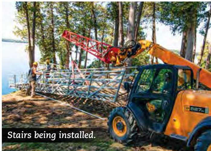
Stair loaded and ready for delivery.
