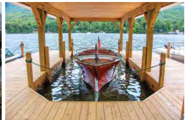
Completed boathouse with crib dock foundation and sundeck.
