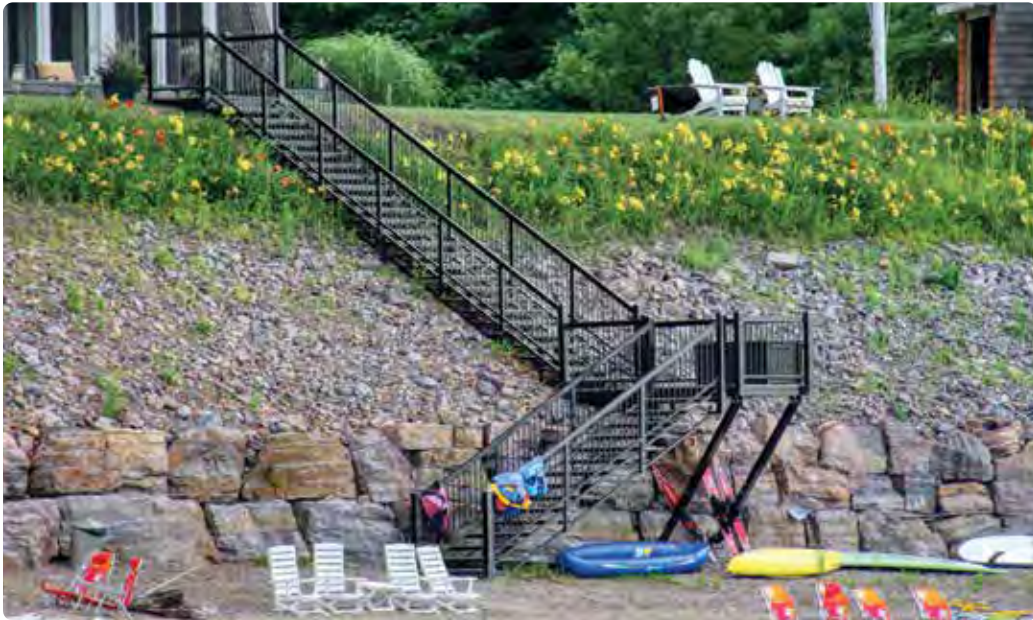
Above: Black powder coated stairs with spindle rail.
