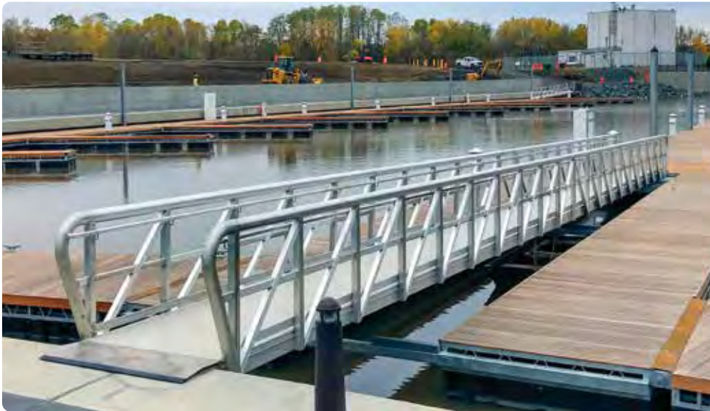
5' x 80' ADA compliant commercial aluminum gangway
