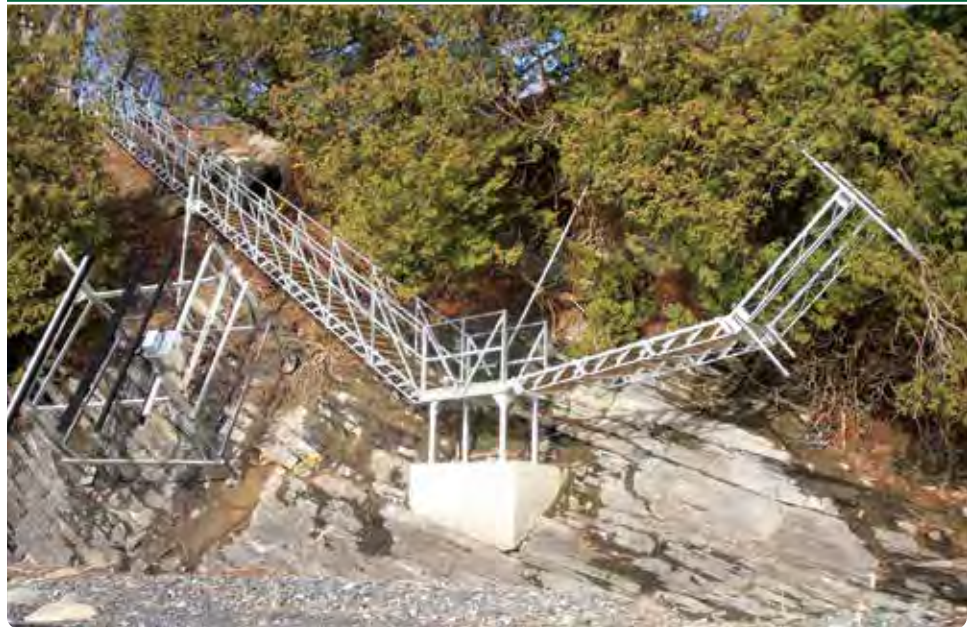
Freespan stairs with lower section that hinges for winter storage.
