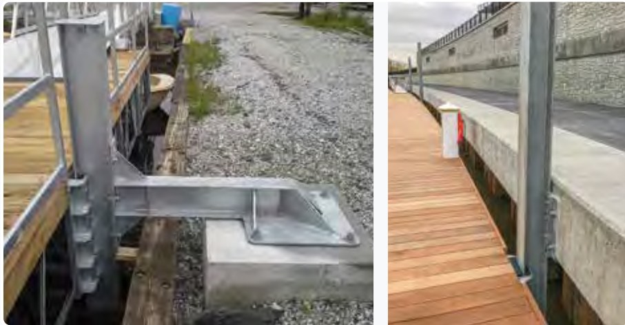
Above: Vertical beam shore mounts.
