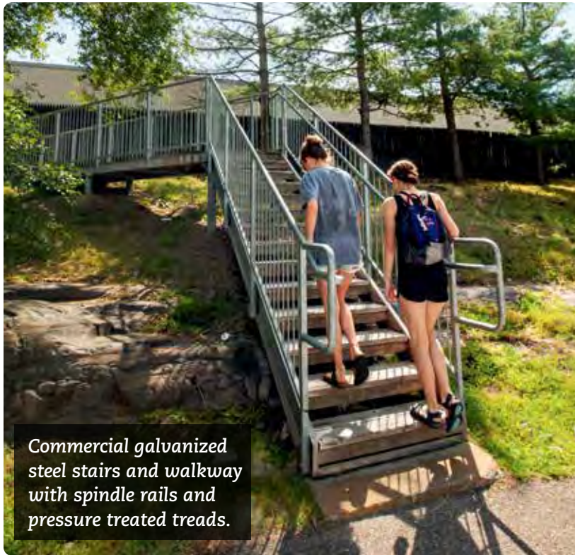
Commercial galvanized steel stairs with pressure treated treads and spindle rails for a children's summer camp.
