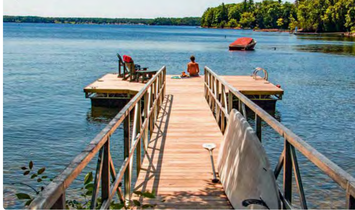
Above: T-shaped floating dock with steel gangway.
