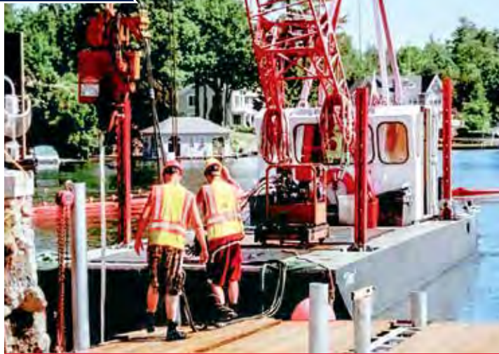
Pile driving from 4" to 12" in diameter (larger if necessary)
