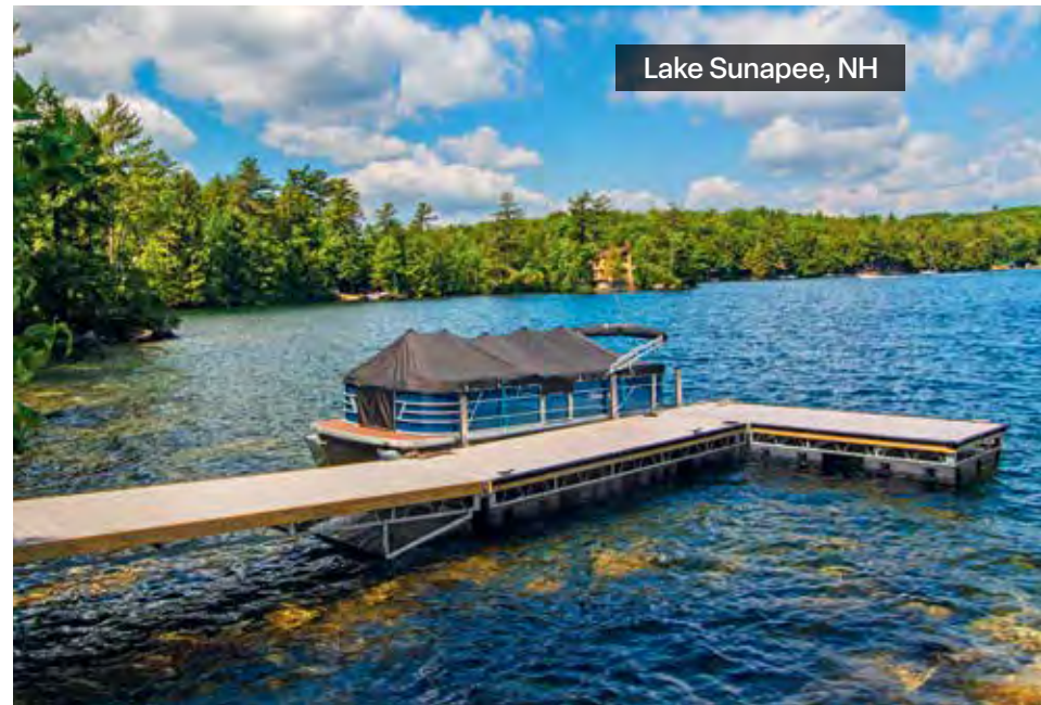
Above: Steel truss floating dock and gangway with Ipe decking. Below Left: Steel truss floating dock with Ipe decking. Our Mega Dock is used as a transition for a site that has high spring water levels. Below Right: L-shaped floating dock with WearDeck decking.
