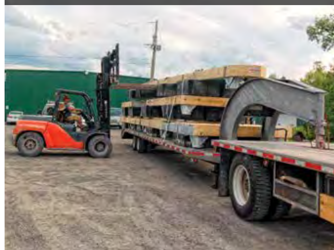
Pile dock sections being loaded for delivery.
