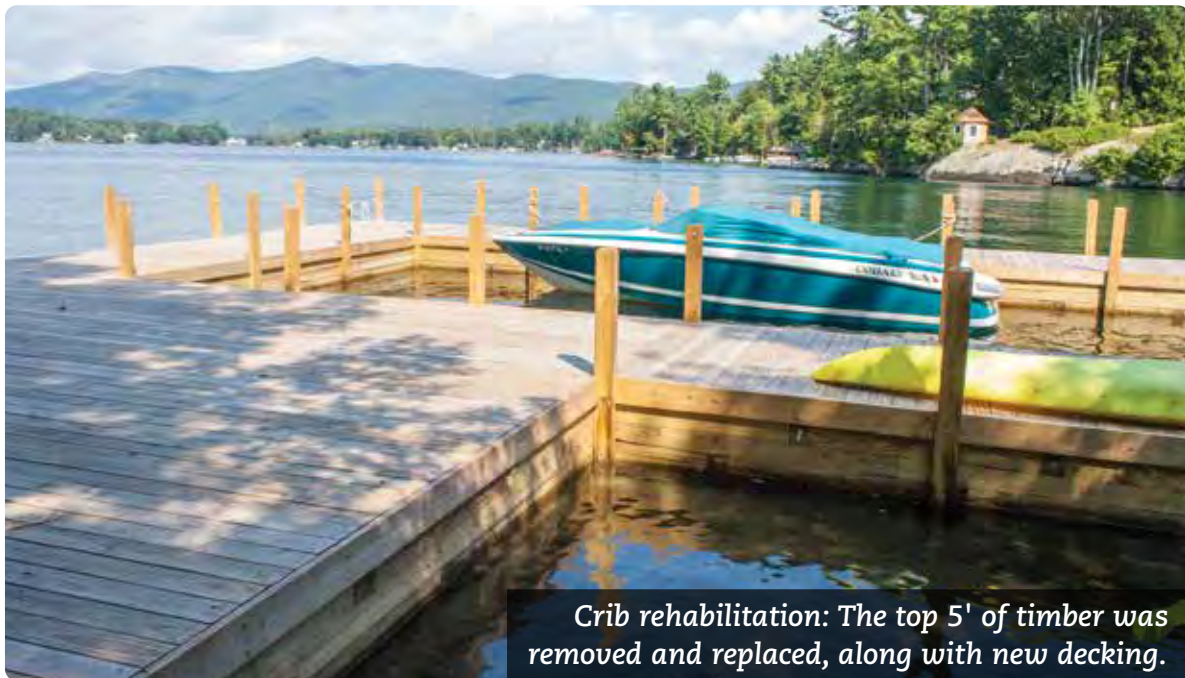
Completed crib dock with rub strakes.
